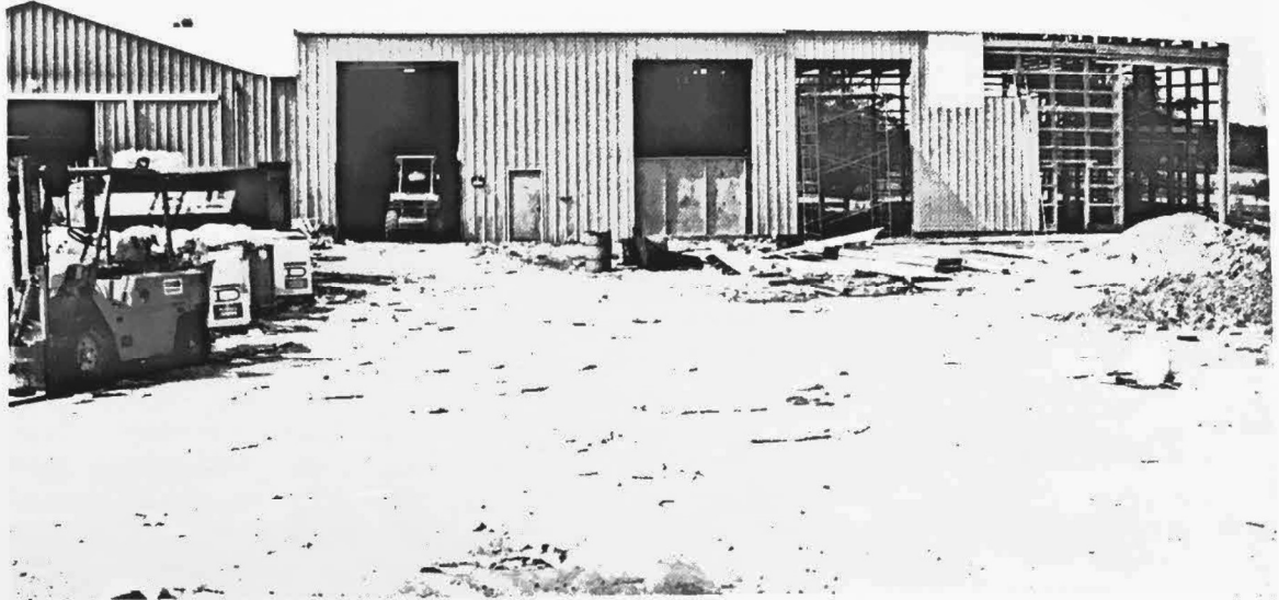
Bigger and Better. An addition is added to the baler building. A new paper baler, which doubles the processing capacity at the site, was recently installed.
